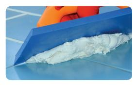
filling in walls is recommended to be made after 2-3 days and in floors after 8-10 days.
